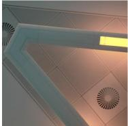
Image of supply diffuser and suspended luminaire
